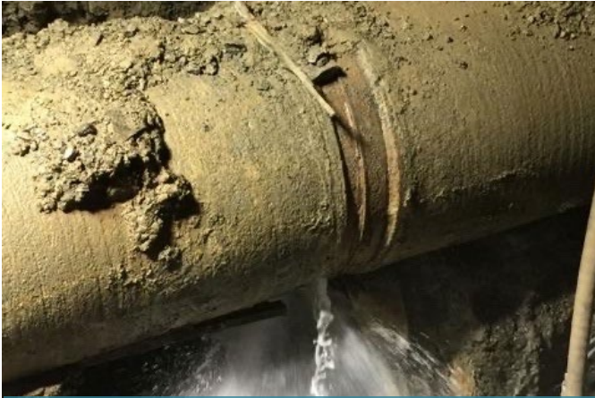
Leak on a 42-in Steel Pipe
