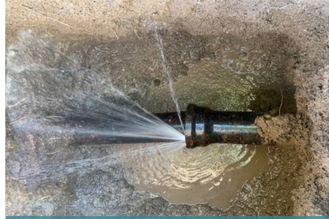
Leak at joint
