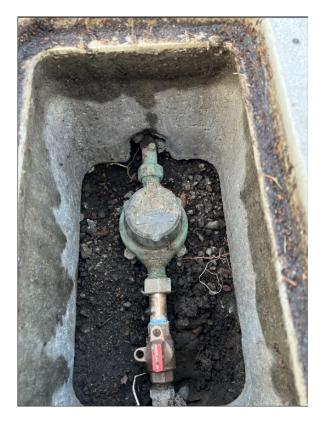
Copper service lines connected to a water meter
