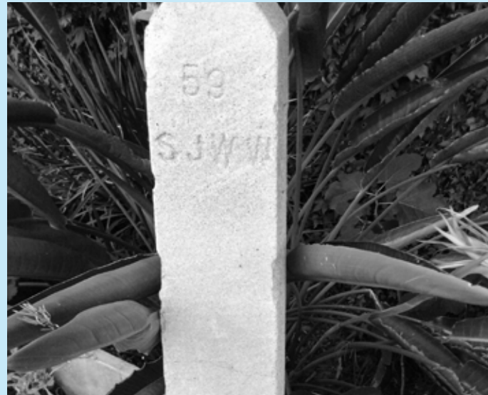
MOUNTAIN METERS – MARKER POST 59, SHOWN HERE, REPRESENTS THE 59TH CUSTOMER TO BE GIVEN SERVICE BY SAN JOSE WATER WORKS.
