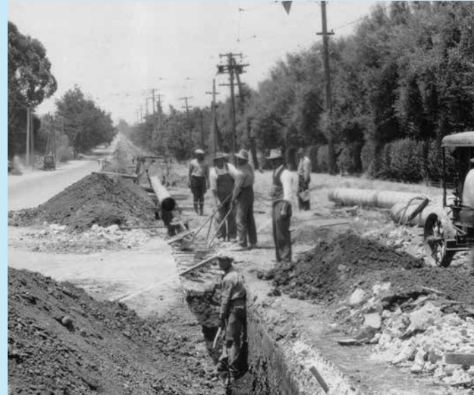
TRENCHES FOR WATER MAINS WERE DUG BY HAND.
