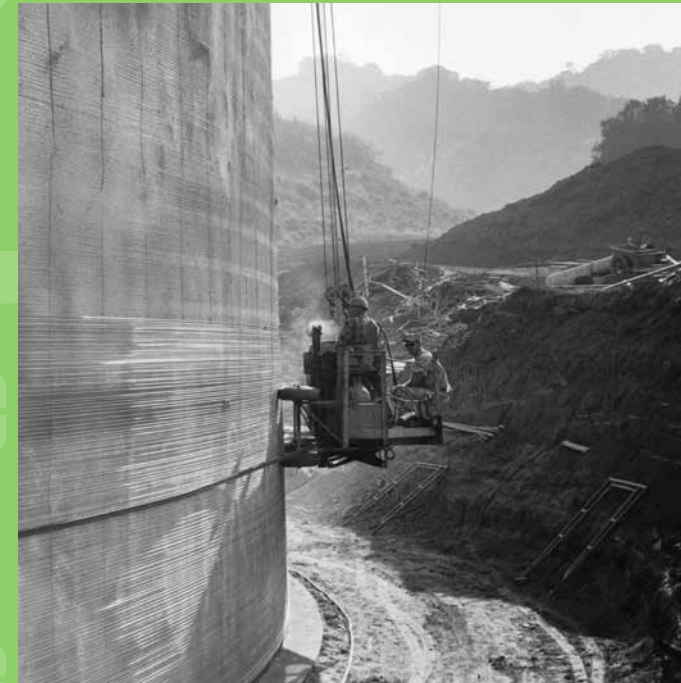
This concrete reservoir in Saratoga, built in 1961, had more than 170 miles of steel reinforcing wire wound around the shell.
