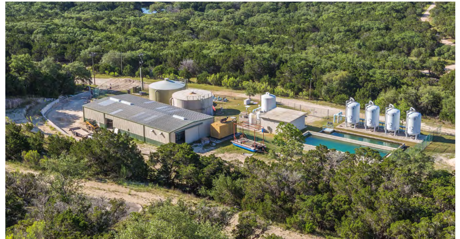
SJWTX water treatment facility
