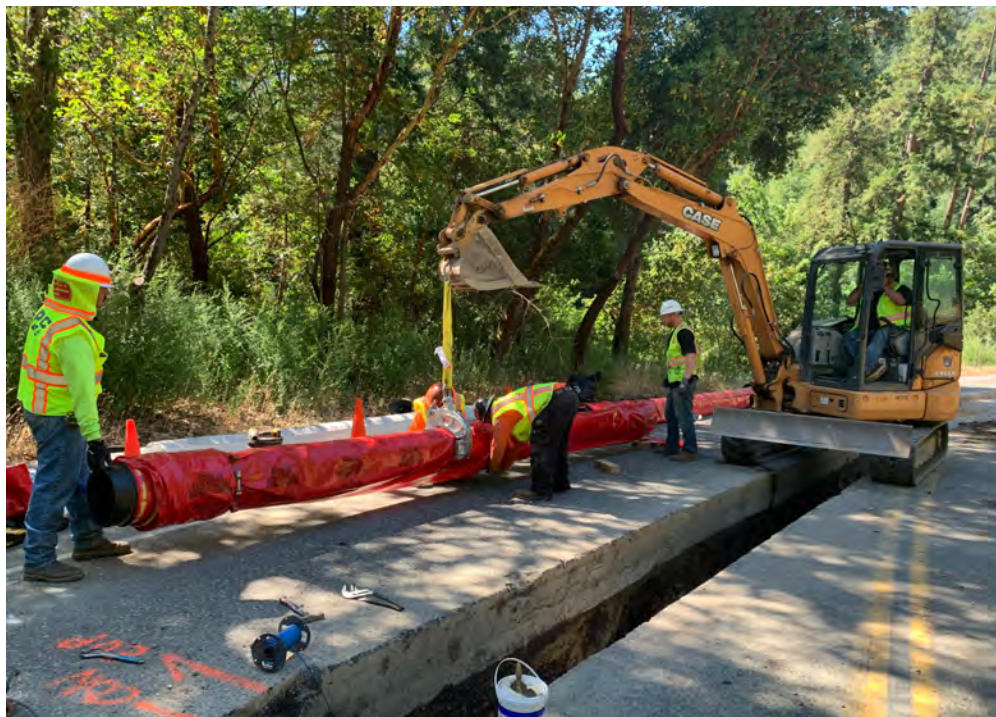
SJW takes seismic safety precautions very seriously and has undertaken a major earthquake-resistant main replacement project in Santa Clara County.
