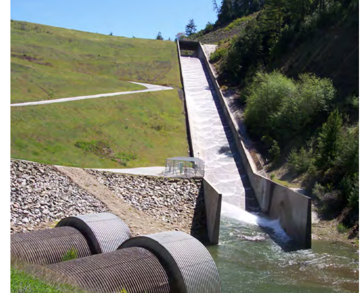
SJW's dam spillway at Lake Elsman in the Santa Cruz Mountains.
