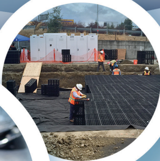
Installing retention chambers for well flushing at Gish Station
