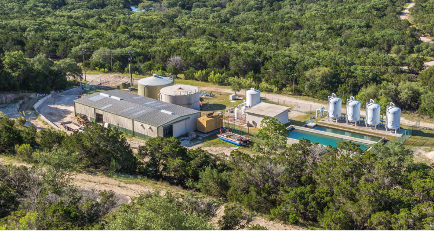
SJWTX water treatment facility
